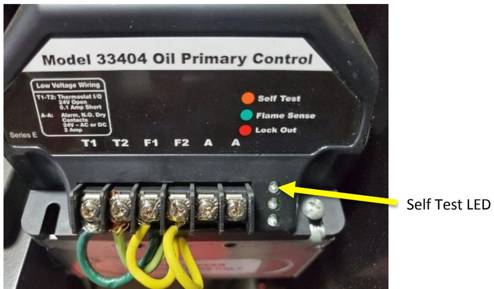
Note: Will blink for a second before the green flame sense light turns no. This simply let's you know the unit has been turned on and will be calling for heat to produce a flame.
