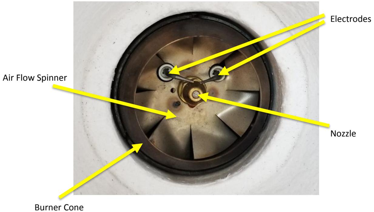
**Note:** It is important that the nozzle and electrodes remain free from excessive build-up. Clean if necessary or replace nozzle. It is critical to never run the unit without the burner cone in place to produce a proper flame.
