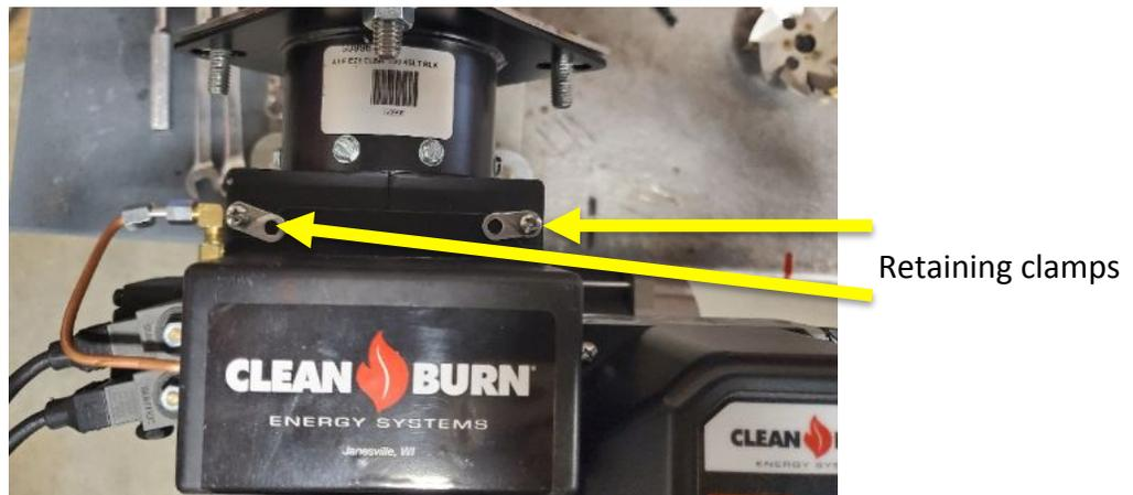
Note: Loosen screws and turn clamps to open igniter assembly.
